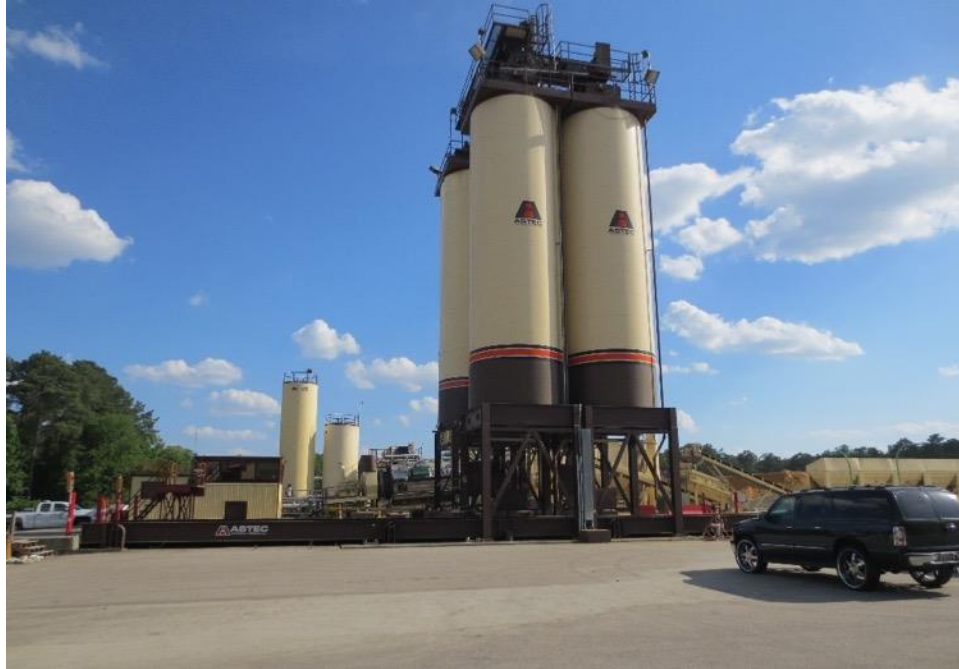
Figure 1. Astec Double Barrel Plant Used in Simms, North Carolina
