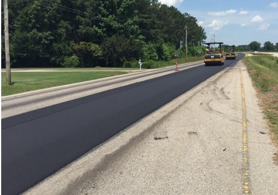
Figure 4. Breakdown and Finishing Rollers Compacting Mat
