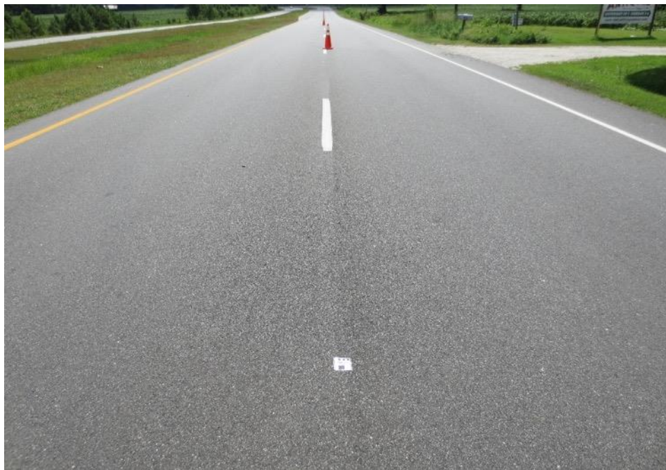
Figure 17. MW RAS HMA (left) and PC RAS HMA (right) at 14-Month Inspection
