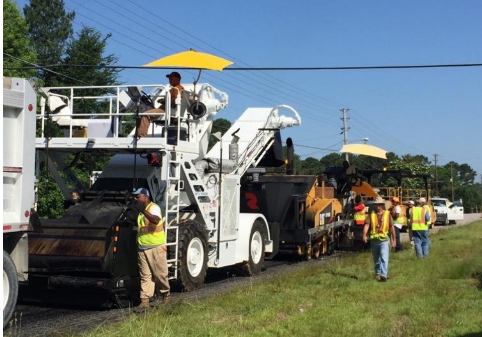
Figure 3. MTV Transferring Mix to Paver
